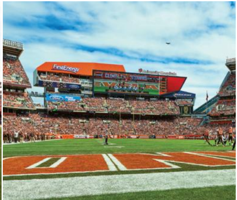
ELECTRIFIED ATMOSPHERE The first phase included major reconfiguration of end zone seating. In the existing east end zone (left), upper level seats were removed and replaced by a new structure (right) with new seating, sponsorship zones and a 6,900-square-foot video screen.
