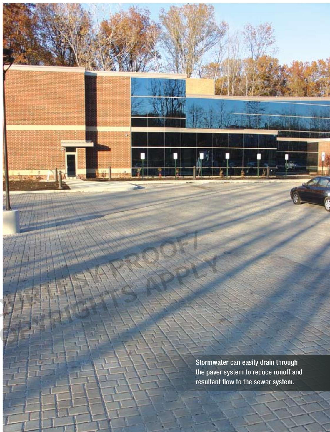
Stormwater can easily drain through the paver system to reduce runoff and resultant flow to the sewer system.
