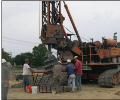
Drilling Caissons
